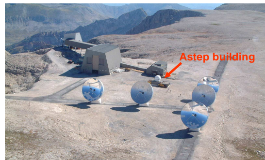
Figure 1. General view of the Observatory on the Plateau de Bure. The ASTEP platform is hosted in Building POM2 indicated in the figure (Photo courtesy of IRAM).
